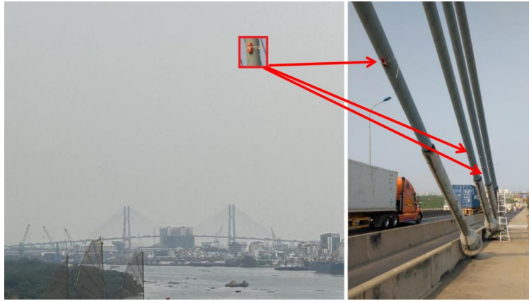
Fig. 2. Vibration measurement on the cables of The Phu My stayed bridge.
